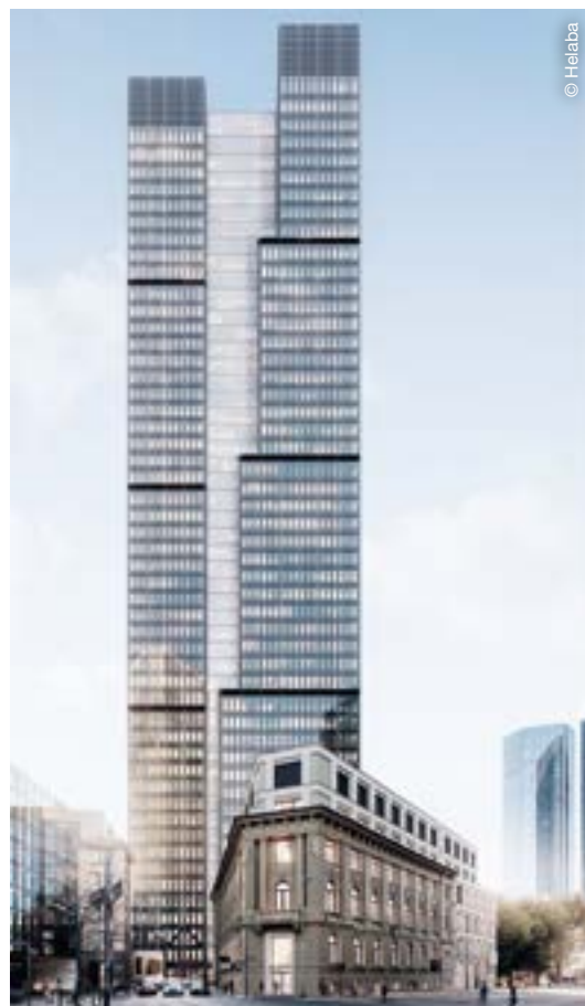
Central Business Tower
