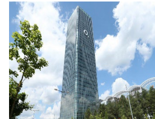
O 2 Telefonica Munich, Germany, Office, data center
