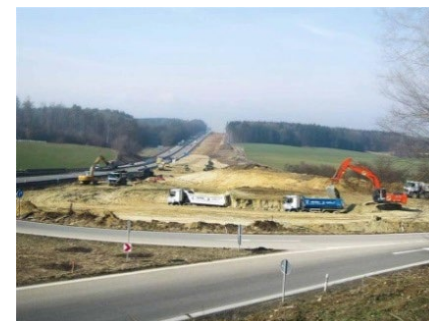
Motorway A8, Germany
