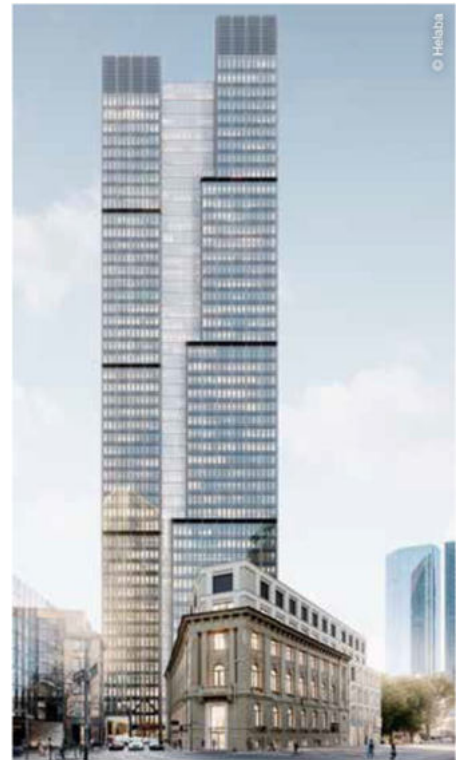
Central Business Tower
