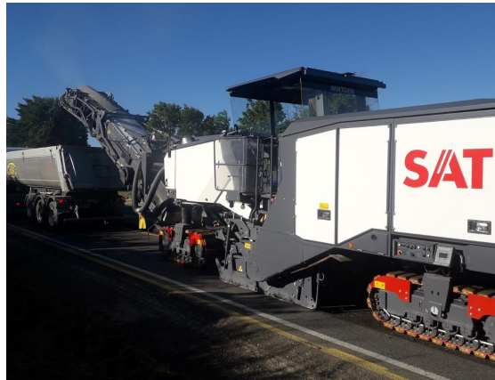
On-site recycling of asphalt
