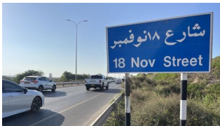
Extensive expansion of 18th of November and Al Mouj streets in Muscat © STRABAG
